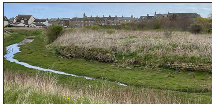
Plans are to raise the surface level of the development as it is in a flood zone. Access will come via Riverside Park.
